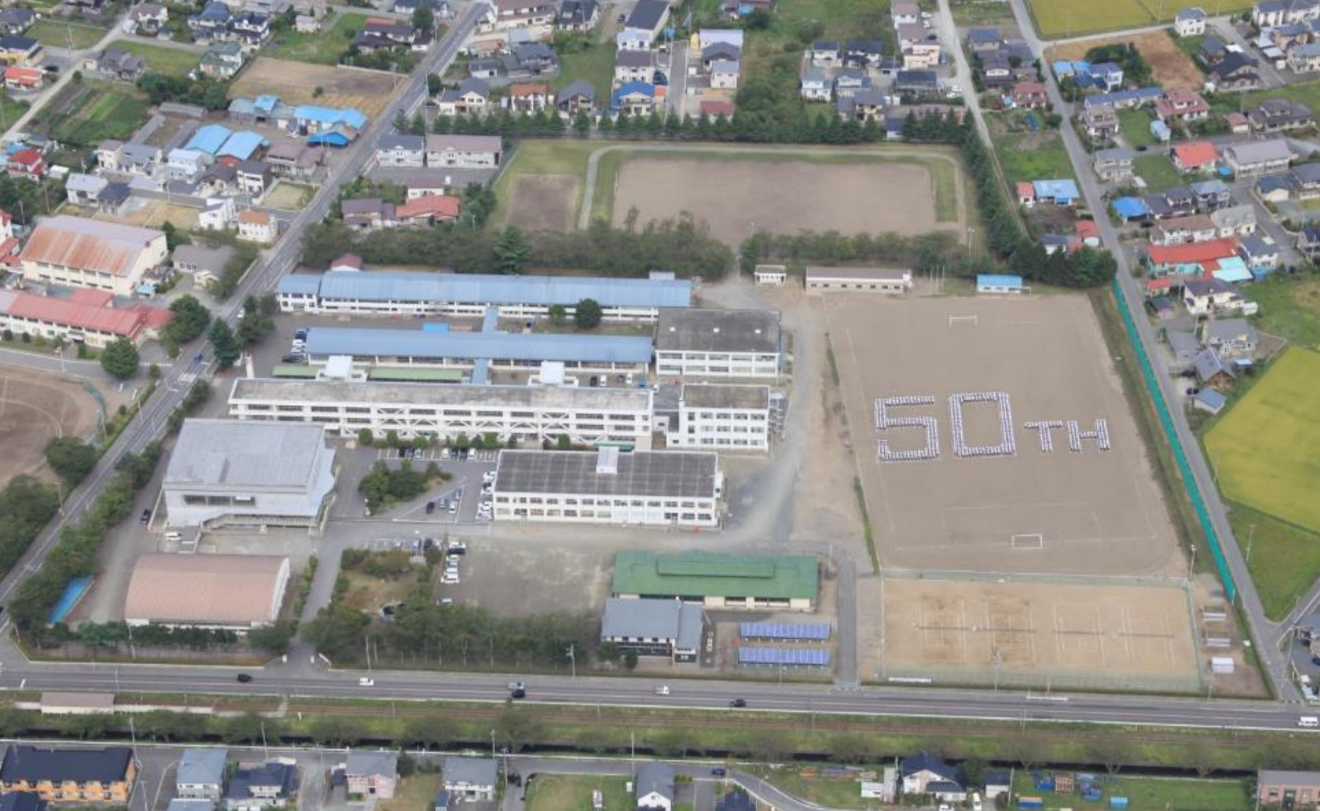
Aomori Prefectural Towada Technical High School
