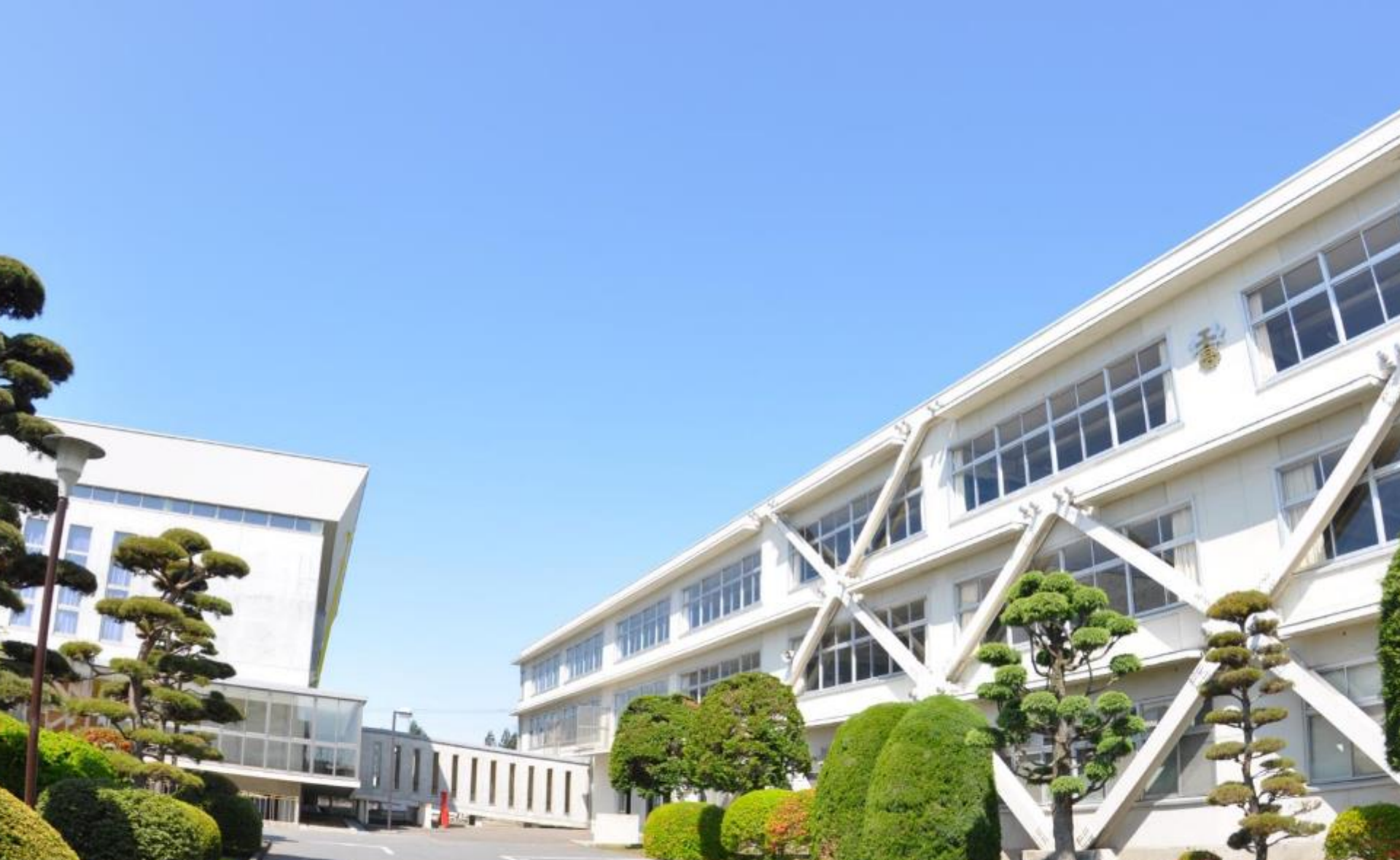
Aomori Prefectural Towada Technical High School
